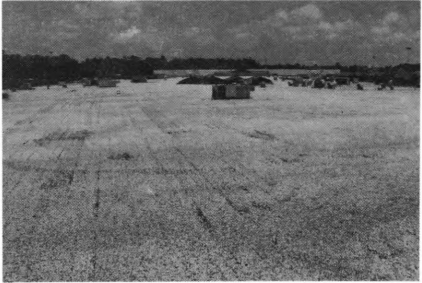
Figure 2. Habitat of roof-nesting Least Terns in New Bern, Craven County, N. C. (Photo by author).
